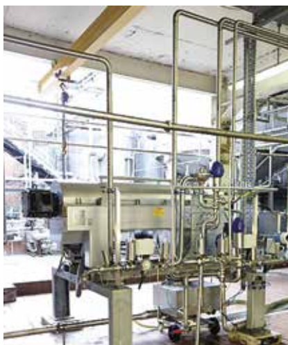
Wort recovery using Foodec decanter centrifuge
