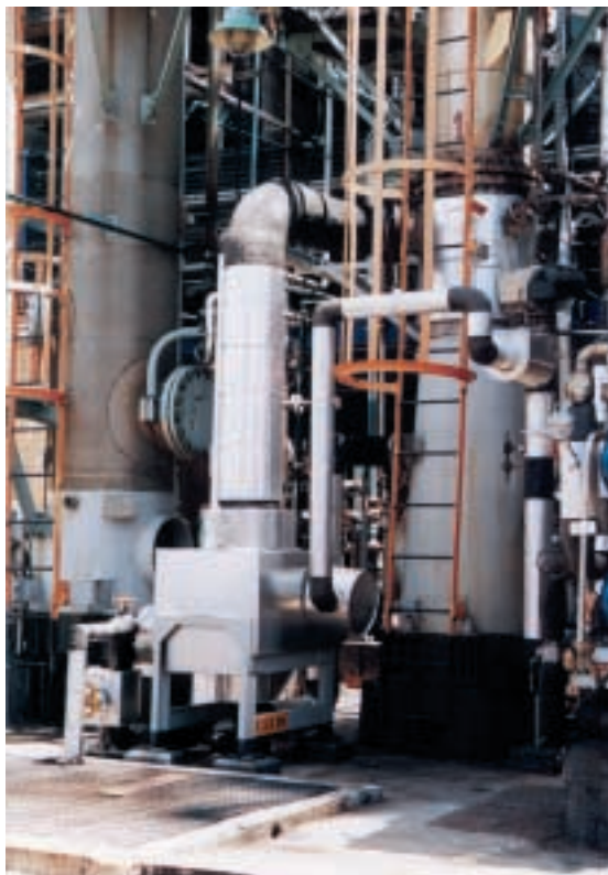
Size comparison: Compabloc versus shell-and-tube reboiler with similar capacity
